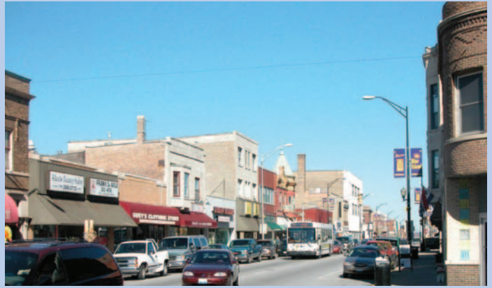
Blue Island's downtown station area includes over 100 businesses and a regional hospital.
