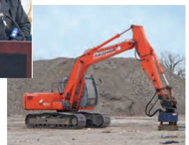
GROUND BREAKING FOR BROWNFIELD CLEANUP AT COD SITE (DIXMOOR, IL)
