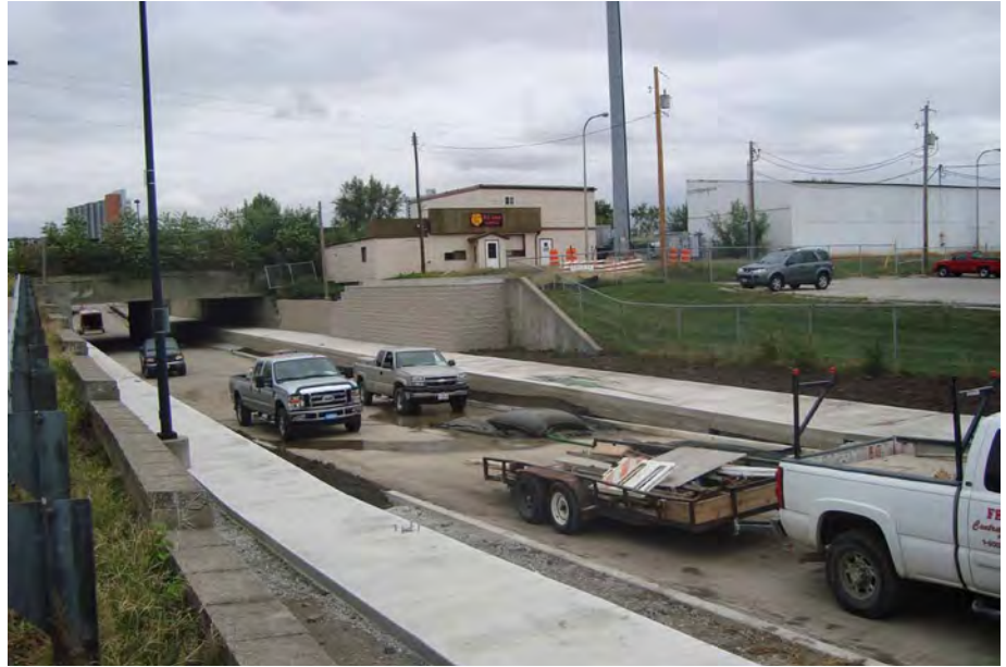
Fig. 9: After On Logan Street at Market looking east during construction
