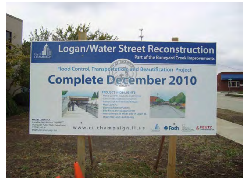
Fig. 67: Improvements such as the Logan/Water Street Reconstruction Project were furthered given the TIF revenue
