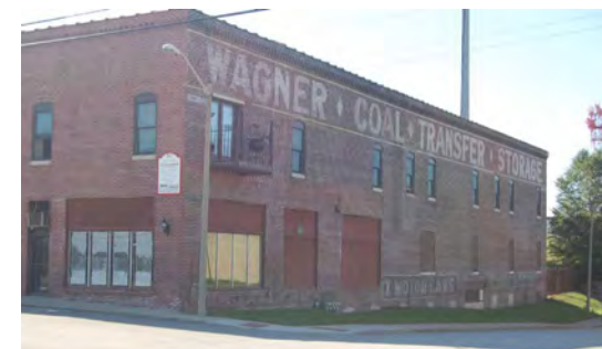
Example of converted warehouse to residential use on White Street
