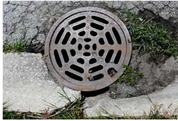
FIGURE RR-6: Degraded Sewer
