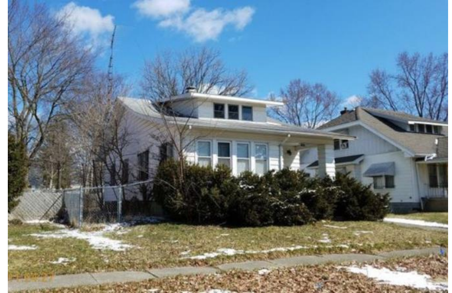
Genesee County Land Bank home in Flint, MI Source: Genesee County Land Bank
