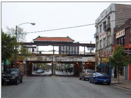
Figure 14. Before and after Argyle streetscaping project. Image: Site Design Group
